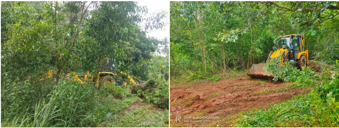
Clearing the land with an earth mover
