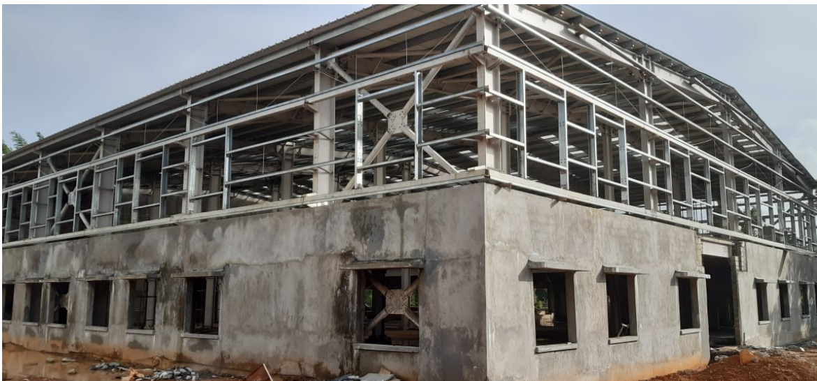
Construction of Training Block on Progress at Technology Centre Angamali
