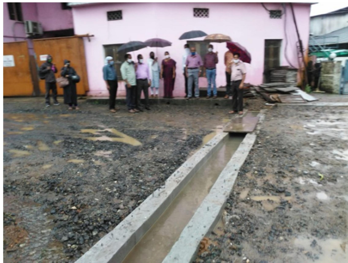
From the Inspection
